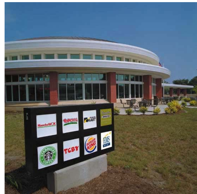
A location on Ohio Turnpike
