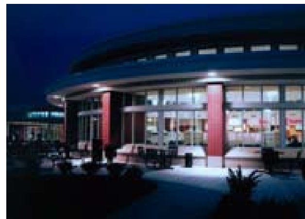
A location on Ohio Turnpike
